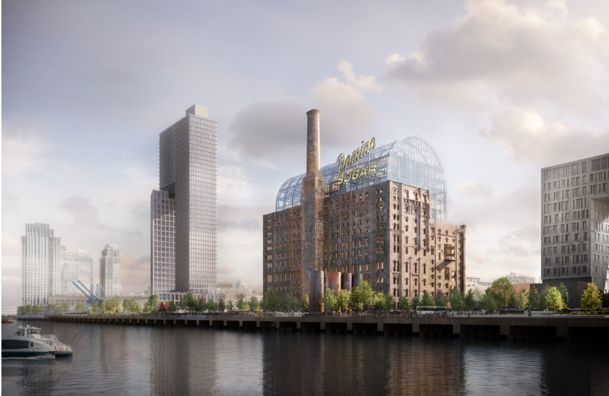
Image 8. PAU was tasked with creating open architecture that seamlessly connects the existing neighborhood to the recaptured waterfront a quarter-mile long. The result is a state-of-the-art, 425,000-square-foot workspace housed within a beautiful, idiosyncratic urban artifact that is unique to post-industrial Williamsburg, offering its inhabitants and the larger community alike a singular experience (image: Courtesy of PAU).
