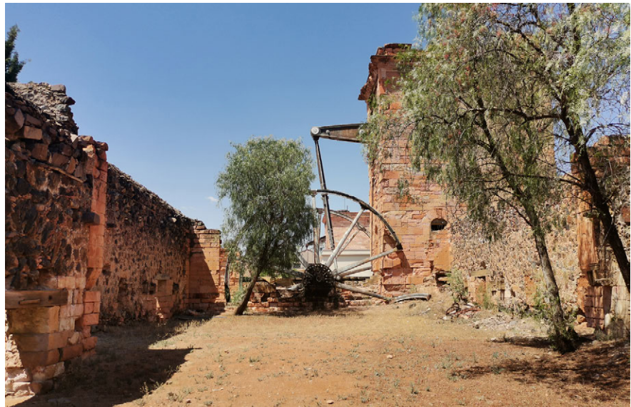
Image 4.- Old Cornish pumps of English technology at Proaño mine, Fresnillo, (source: Authors' own, 2024).
